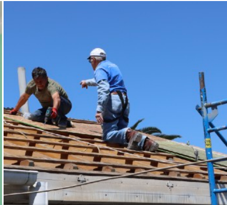
Replacing the roof
